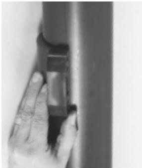
1. Position lower half of saddle around pipe.
