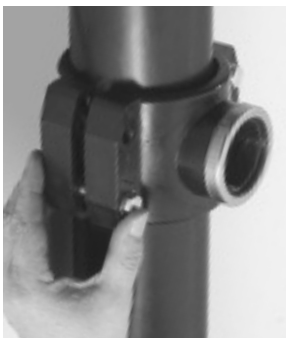
2. Taking care to seat gasket, bolt both halves together.
