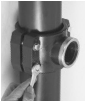
3. Use a spanner to tighten. Do not over torque!
